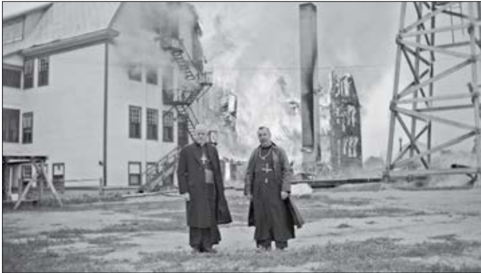
The Roman Catholic school at Sturgeon Landing, Saskatchewan, was destroyed by fire in September 1952. There was no loss of life. St. Boniface Historical Society Archives, Roman Catholic Archbishop of Keewatin-The Pas Fonds, N3637.
